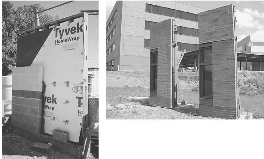
Figure 17-5 Masonry mock-ups should include all elements important to the performance and appearance of the masonry such as backing wall, anchors, drainage mat, flashing, weeps, movement joints, and windows.
